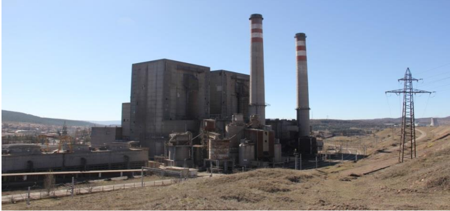
Tunçbilek Termik Santrali
